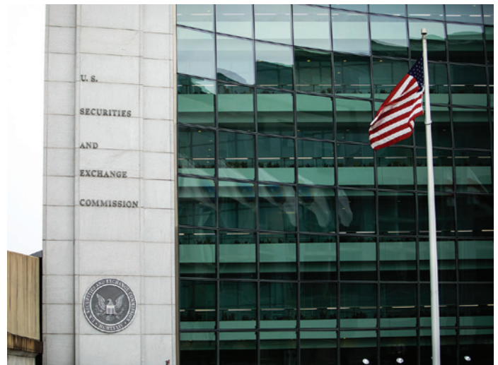
U.S. Securities and Exchange Commission building in Washington.
